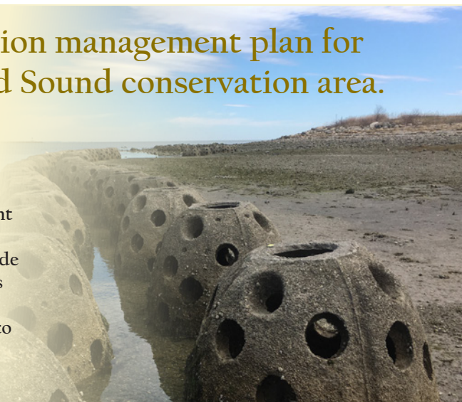
Rows of 'reef balls' form an experimental storm barrier along the shoreline of Stratford Point, CT. This artificial reef provides physical protection for the site's eroding shoreline and creates opportunities for shellfish to recolonize the area.
